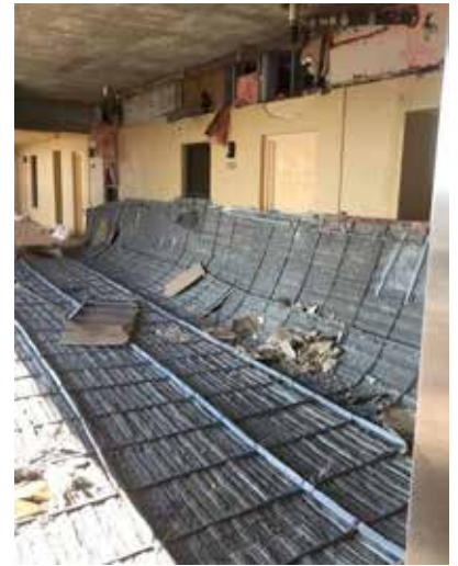
Ceiling smashed to the floor, beside tower elevators.
