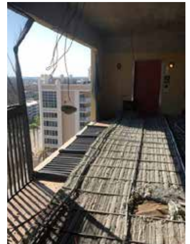
10th floor corridor -- broken-down railings, screens gone, cracked walkways.
